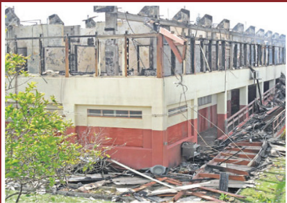
Gutted by fire in 2009
